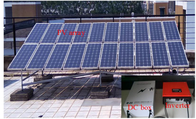
Fig. 16. Photograph of a 3 \times 6 scale PV system.
